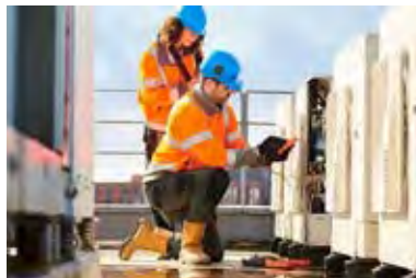
Building Training Programs for Maintenance Staff
